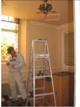
Mr. Machen remodeling Bride's Room/Office
